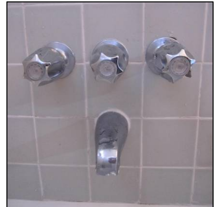
Figure 1: A diverter valve as part of a three-handle shower valve
