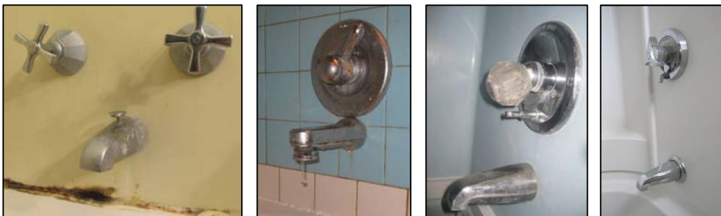
Figure 2: Examples of plate diverters. From left to right: a lift on the tub spout diverter with a two-handle valve; a pull-down ring on the tub spout diverter with a single-handle valve; a button on the valve plate with a single-handle valve; and a sliding lever on the valve plate with a single-handle valve.
