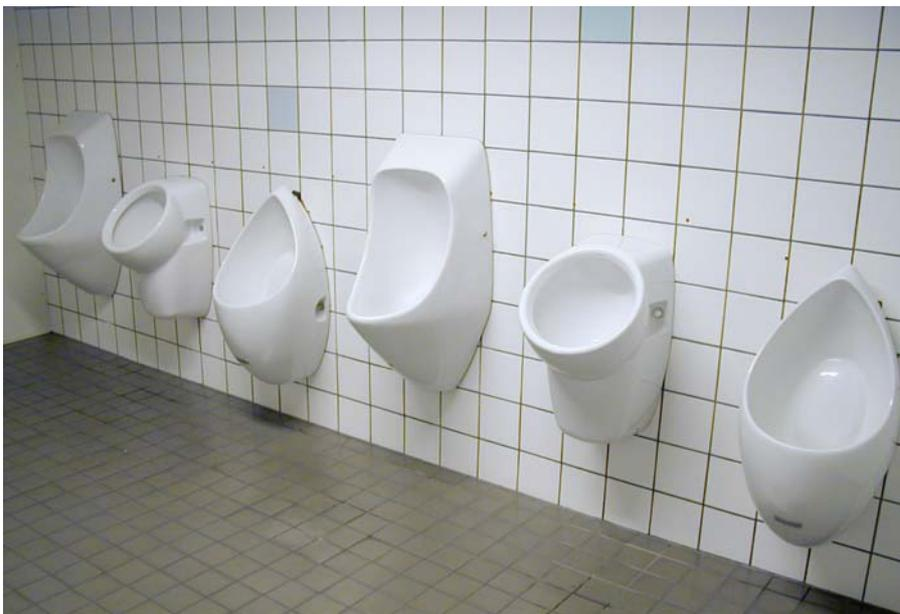
Figur 5: Test Dry Urinals (from r.to l.): Urimat, Sphinx, Mc Dry (Duravit)
