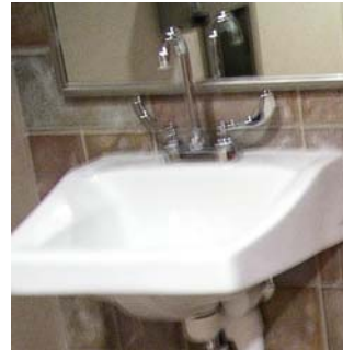
Existing Faucet – handicap stall
