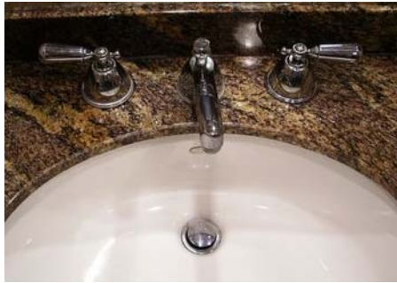
Existing Faucet – general area
